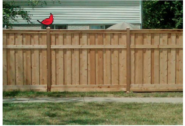
6' Tall Custom Board & Batten with Custom Trim
