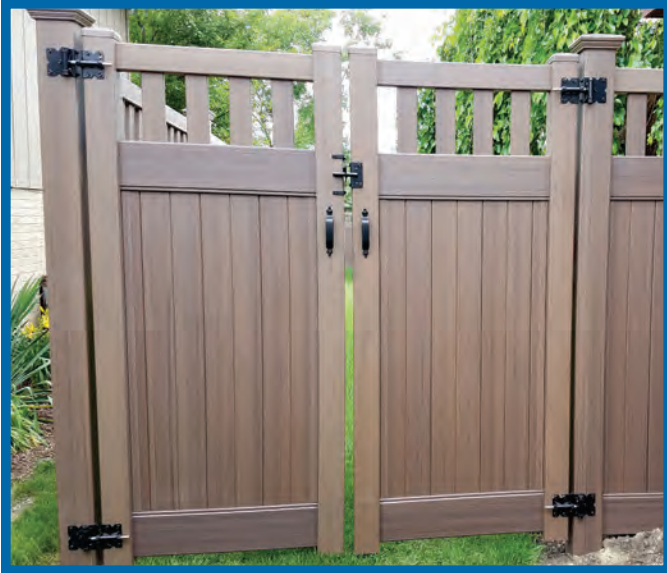
Drop Rods Are Installed On The Inside Face of Double Gates
