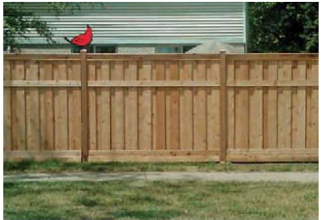
6' Tall Custom Board & Batten with Custom Trim
