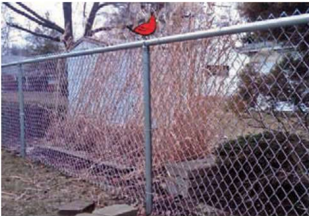
4' Tall Galvanized Chain Link Inside View
