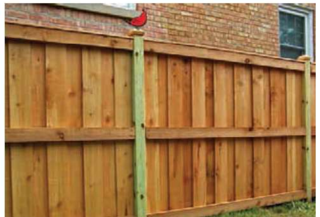
6' Tall Board on Batten with Top Cap, Trim Boards and Treated Posts - Inside View
